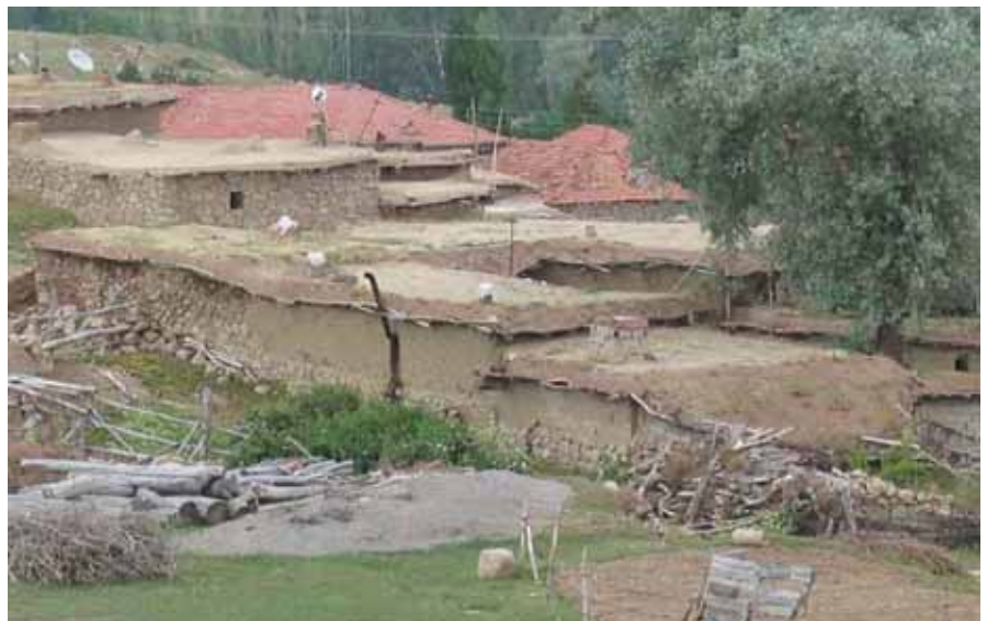
Figure 4. This village still has a number of typical traditional mudbrick and flat thatch roof complexes that have not become hybrids with newer gabled roofs yet, though each home has a protruding television antenna dish (A. Snyder, 2002).
