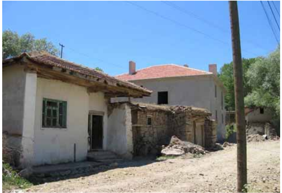
Figure 5. One type of hybrid existence is the saved older mudbrick or stone structure sitting next to a new, oversized, free standing, in-filled concrete frame structure (A. Snyder, 2002).
