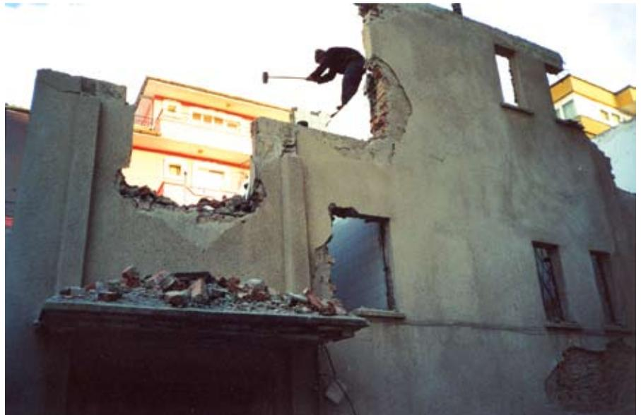
without fall-protection and the worker is demolishing the very wall on which he is standing.
