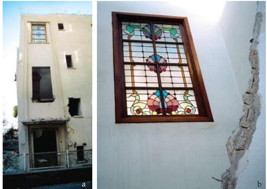
**Figure 1.** Stained glass windows of a building on Farabi Street in Ankara, that was demolished: (a) the lower window was dismantled but the one on top was discarded for lack of appropriate rig; (b) close-up of the window from inside the stairwell.
