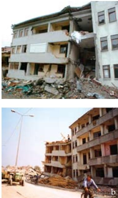
**Figure 4.** (a) A building damaged severely during the August 1999 earthquake in Adapazarı. (b) The building has been stripped of any reusable building material (doors, windows, tiles); and timber from the roof is being salvaged.
