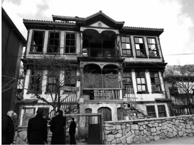
Figure 5. Delegation from İzzet Baysal University in front of Haytalar Mansion, Mudurnu, which the university planned to take over for restoration and reuse (photo: E. Yıldırım, 2009)
