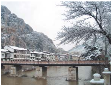
Figure 5c. Eastern bridge raised on the remains of a Roman bridge (Aydan Balamir).
