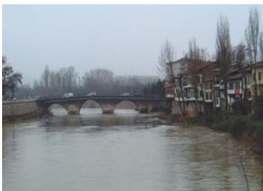
Figure 5d. Western bridge (Aydan Balamir).
