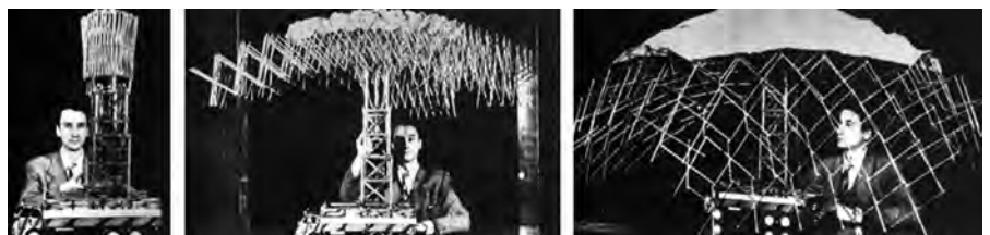
Figure 15. Pinero’s scissor mechanisms for deployable structures (Robbin, 1996).
