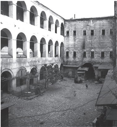
Figure 10. View of courtyard galleries and later addition in rough stone that divides the han's courtyard into two (Nicholas V. Artamonoff Collection)
