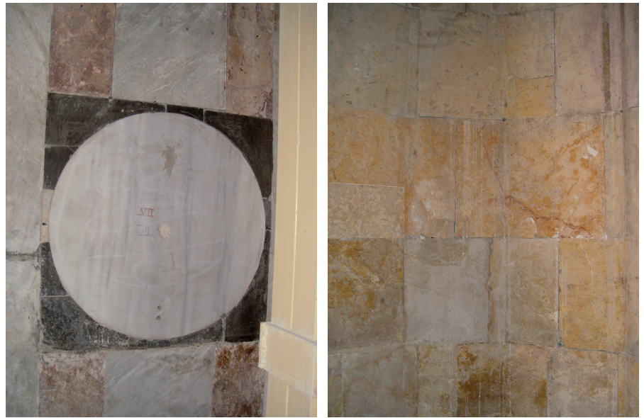
Figure 31. Holes for injecting mortar on the interior walls of Süleymaniye Mosque, 2005
