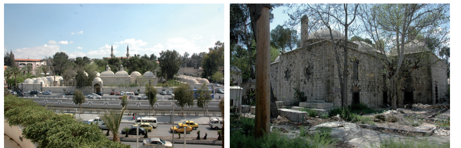
Figure 18. Imaret a) View from north, the Caravanserai masses on sides, b) View from the inner garden in the north-eastern corner, 2009.
