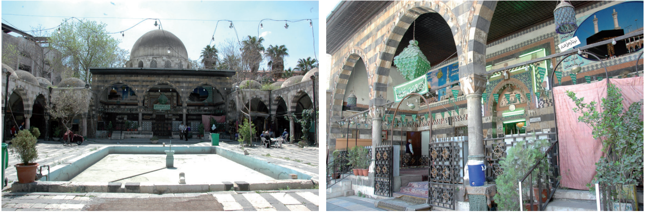
Figure 22. a) View of the Classroom of Madrasa and the pool at the courtyard from the entrance, b) View of portico in front of the Classroom from west, 2009.
