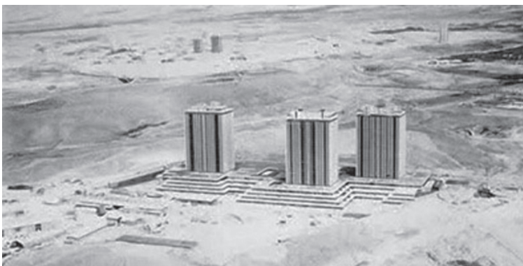
Figure 10. Eskin towers under construction, street view, Tehran, 1976 (Honar-e Memari, 2020)
