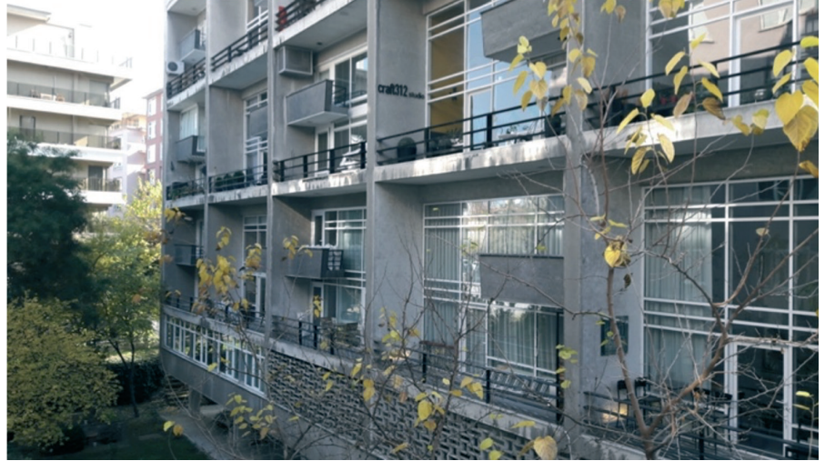
Figure 6. The north façade of the Cinnah 19 Apartment (Authors, 2022).
