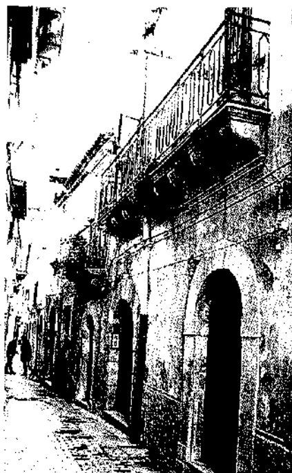
Figure 24. Ortigia survey of houses, house number 14 (photograph by author).
