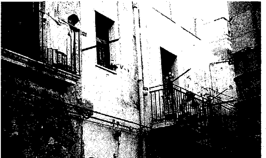
Figure 20. Ortigia survey of houses, house number 20 (photograph by author).
