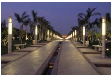
Figure 11a, 11b. Lights and lighting system: while designed to achieve dramatic visual effects in aesthetic terms, it was a source of users' dissatisfaction in functional terms. (Gary Otte, AKTC, Geneva).
