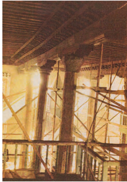
Figure 7. Ahi Elvan Camii maintenance and repainting campaign in 1970s (VGM Archives).
