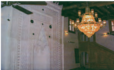
Figure 15. Örtmeli Mesjidi cast stucco mihrab after restoration (Photo: E. Erder).
