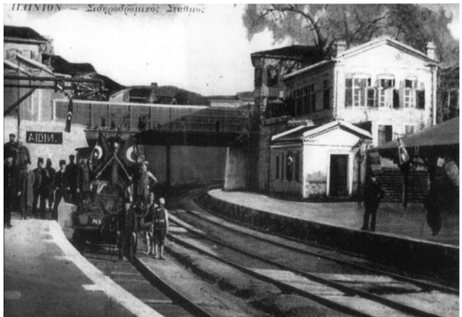
Figure 6. A postcard (ΑΙΔΙΝΙΟΝ - Σιδηροδρομικός Σταθμός) showing the Station Bridge in 1900s (Ünlü, 2007).
