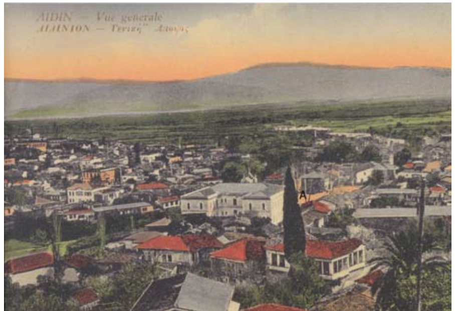
Figure 8. A postcard ( Aidin – Vue generale , ΑΙΔΙΝΙΟΝ - Γενική Άποψη) showing the Government Building and its surroundings. A. Governmental Plaza (Ünlü, 2007).
