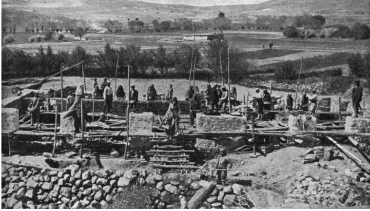
**Figure 1.** The villagers working at a school construction (Köy Okulu Binası, 1937). Close examination of the photo reveals that women also worked at constructions. Right in front of the building, a woman is mixing mortar with a shovel, and other women are carrying construction materials to the building and other places as needed.
