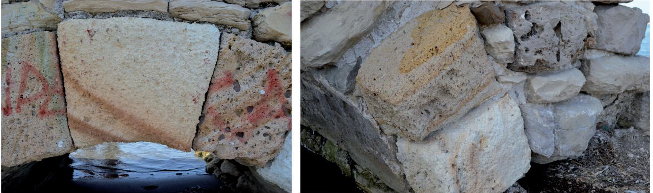
**Figure 9.** Lime mortar connecting voussoirs with each other and spandrel wall
