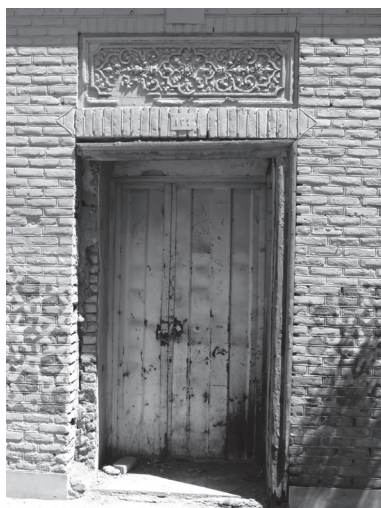
Figure 7. Chamran St. House in Mashhad, brick decoration on the main façade (from authors archive, 2016).
